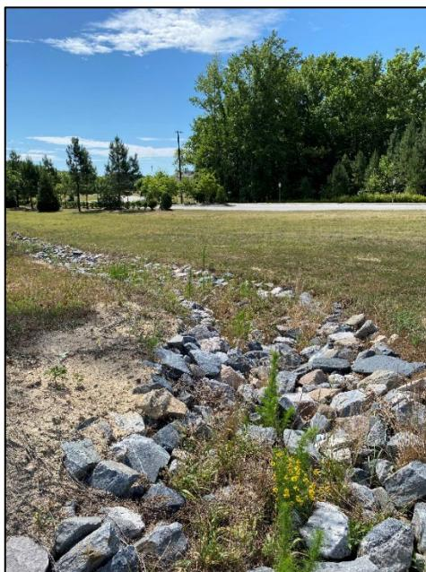
Figure 1. Example of rip-rap lining eroding channel downslope of pipe outlet
