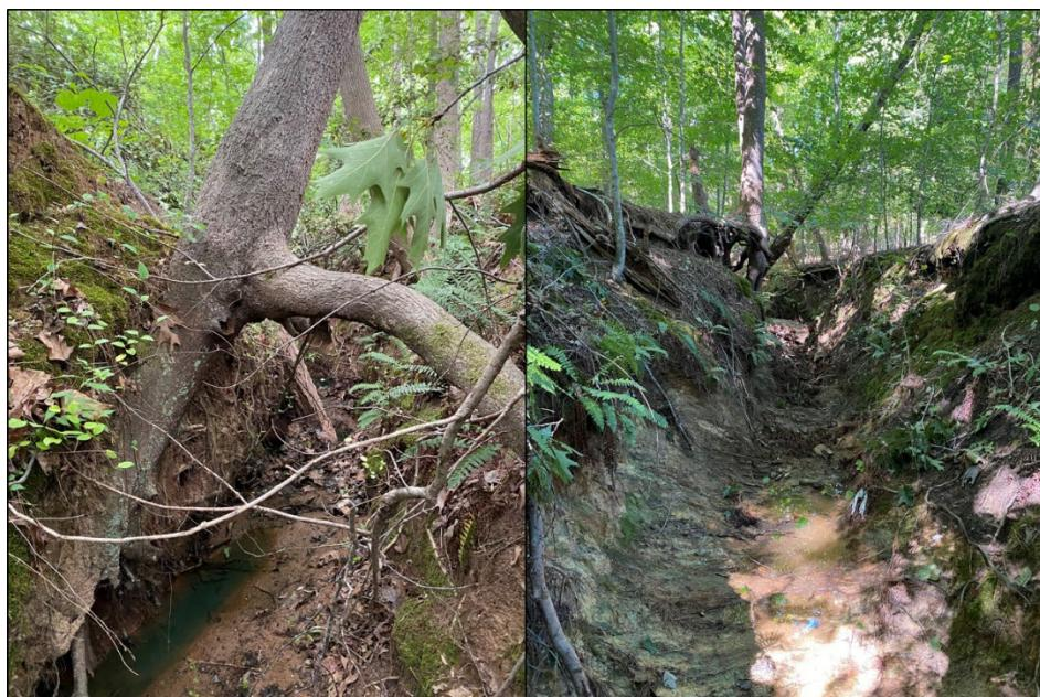
Figure 2. Examples of gullies downslope of pipe outlets
